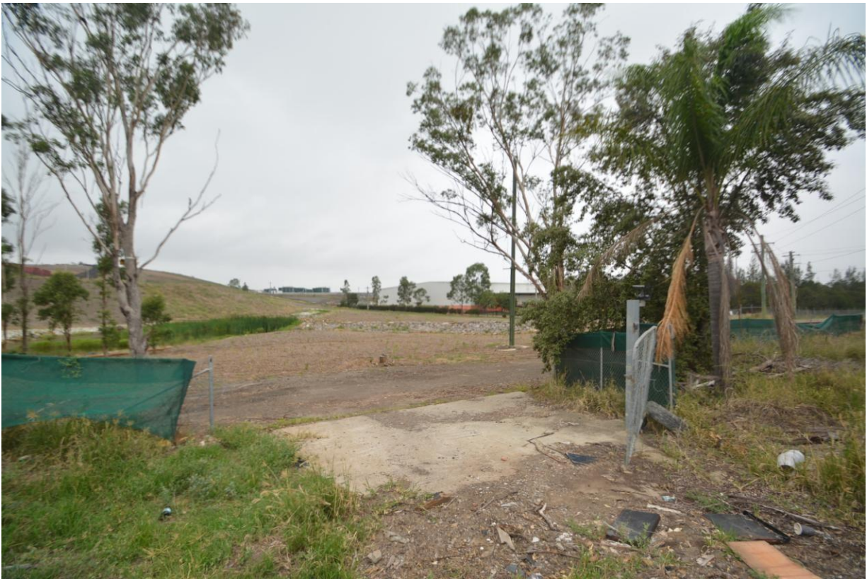
View of site from Erskine Park Road
