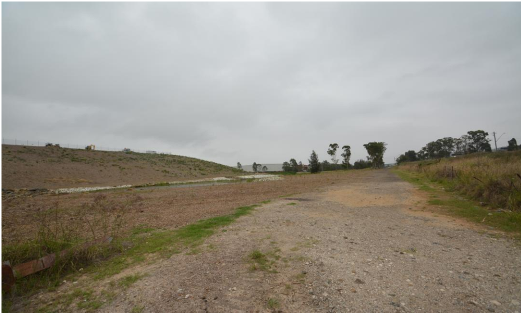
View of southern boundary and adjoining creek and rehabilitated green corridor
