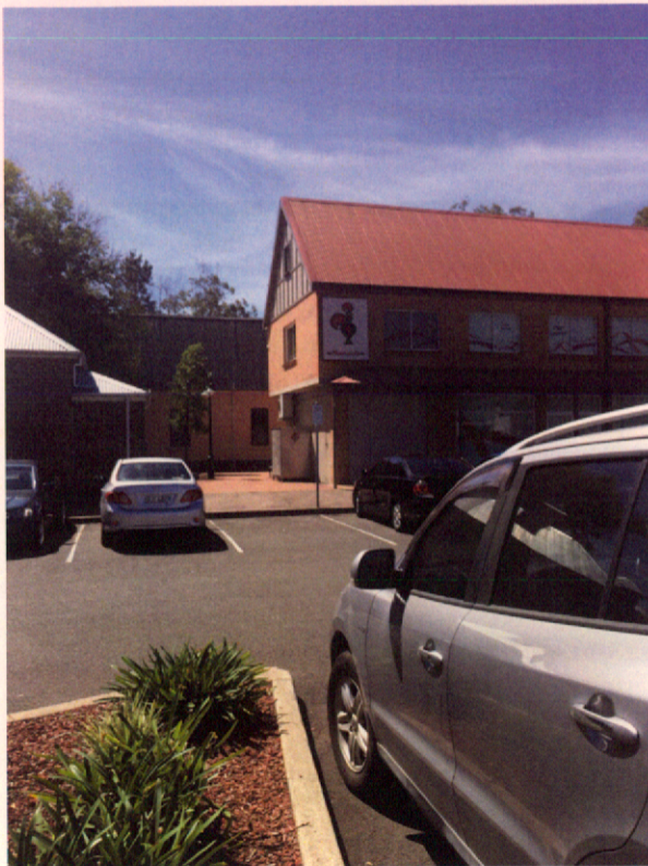
Image 1 – View of shop suite H006 and H004 from car park
