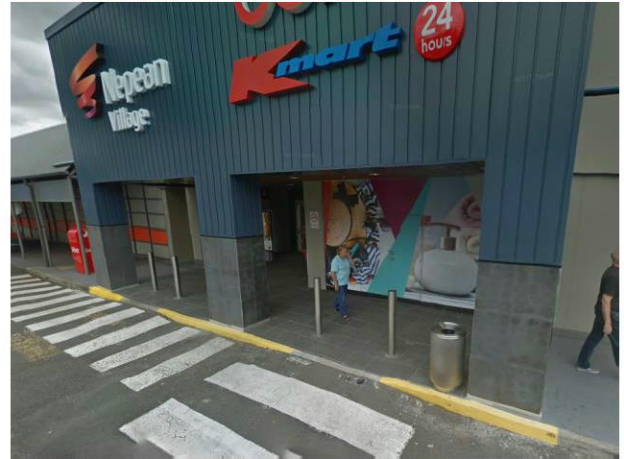
Figure 7: External view of tenancy
