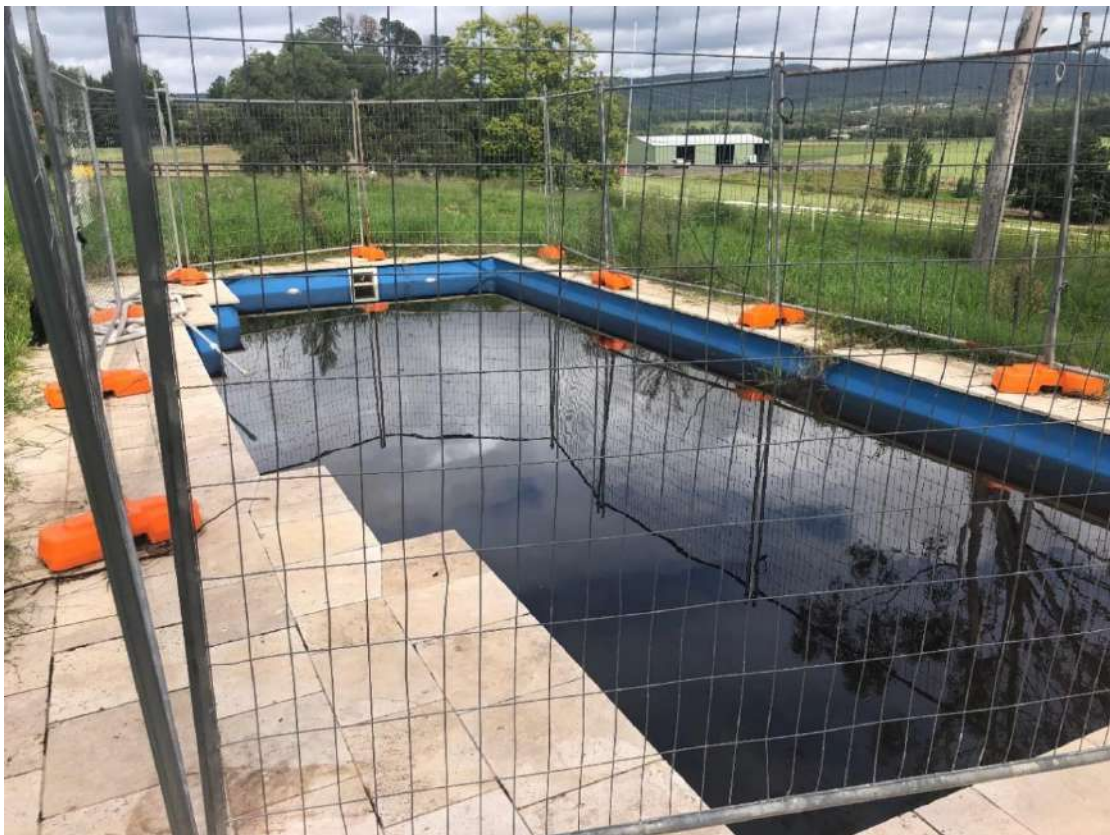
Photo 4: Decommissioned pool looking north
