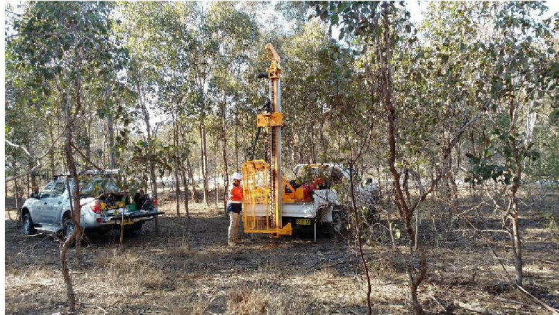
Figure 2 – AG's investigation - drilling BH501
