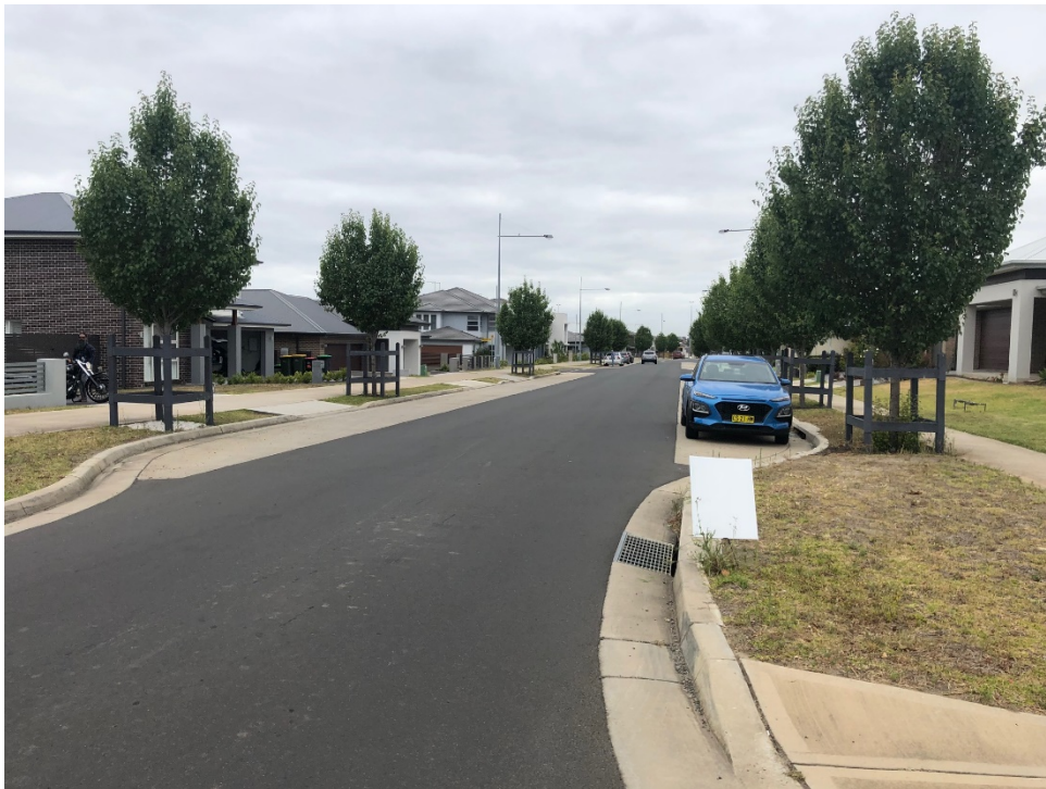
Figure 4a: Bradly Street facing East
