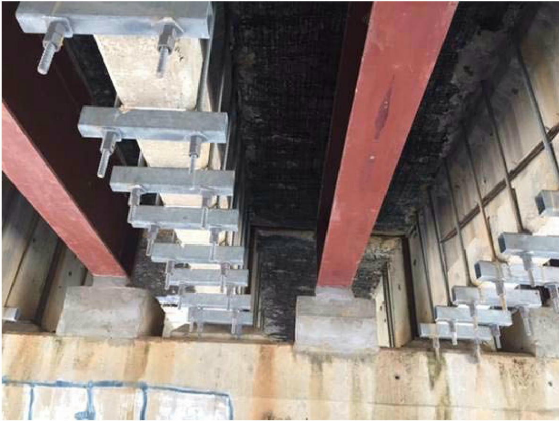
Photograph 3 View of the underside of Ropes Creek Bridge
