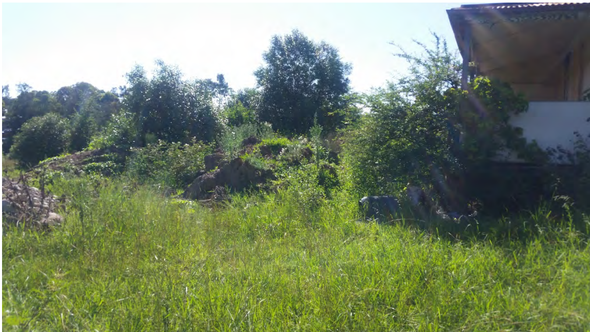
Shed on Lot 3 behind residence, facing South – 11/03/20
