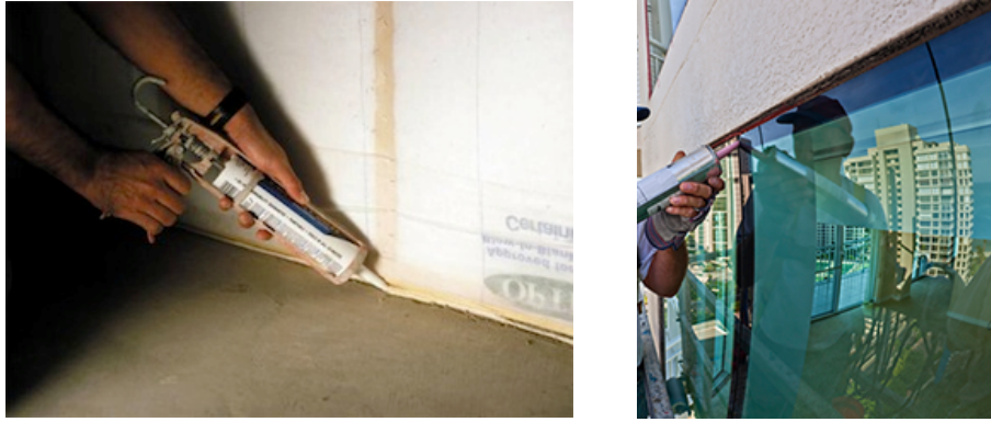
Figure 8 interior and exterior building sealing
