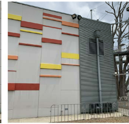
Existing pre-cast concrete panels with feature colour panels to be retained. Existing corrugated cladding to be retained.
