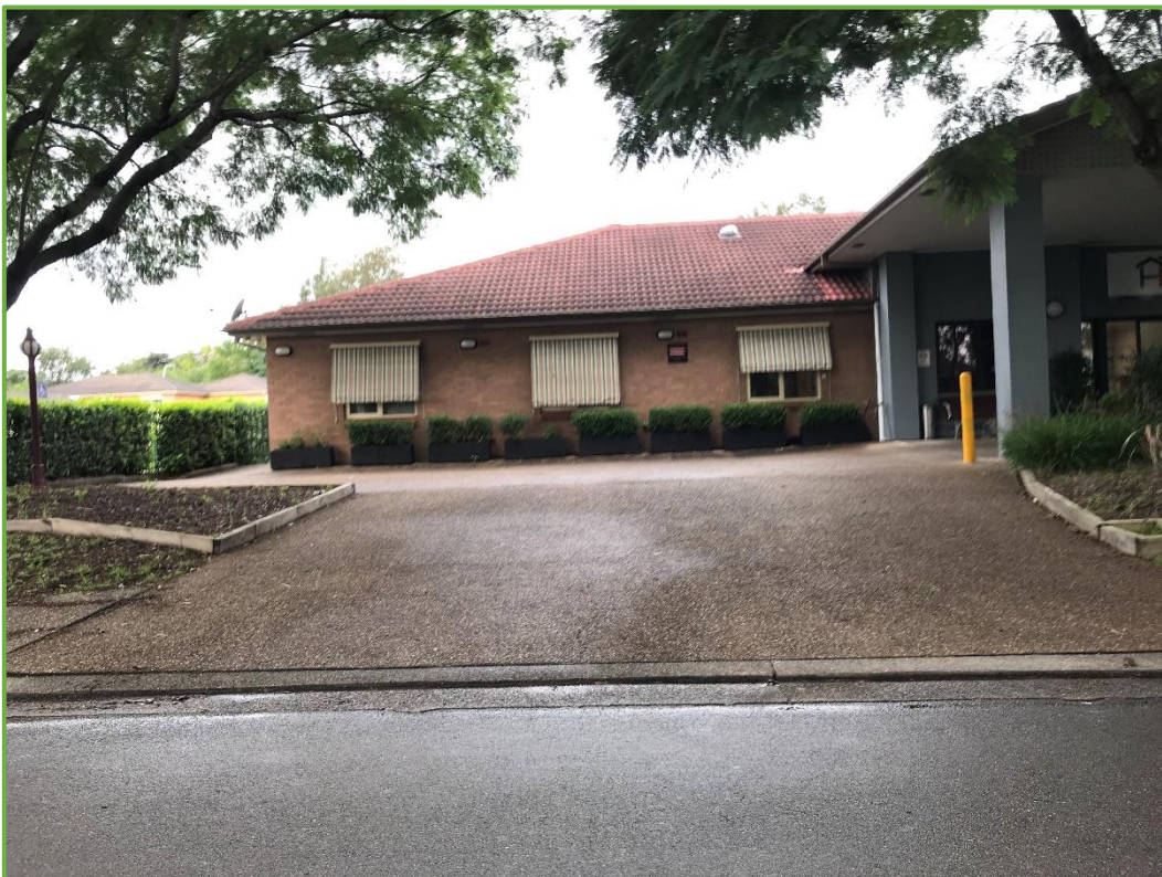
View looking east across Mulgoa Road, towards the subject site's northern access driveway
