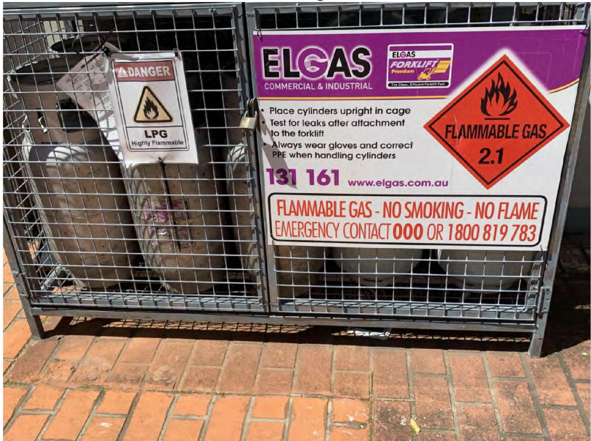
Photograph 8: Locked cage holding Liquefied Petroleum Gas (LPG) tanks was located at the rear of Building 3.
