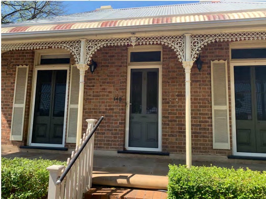
Photograph 1: Building 1. 148 Station Street, Penrith. Currently vacant.
