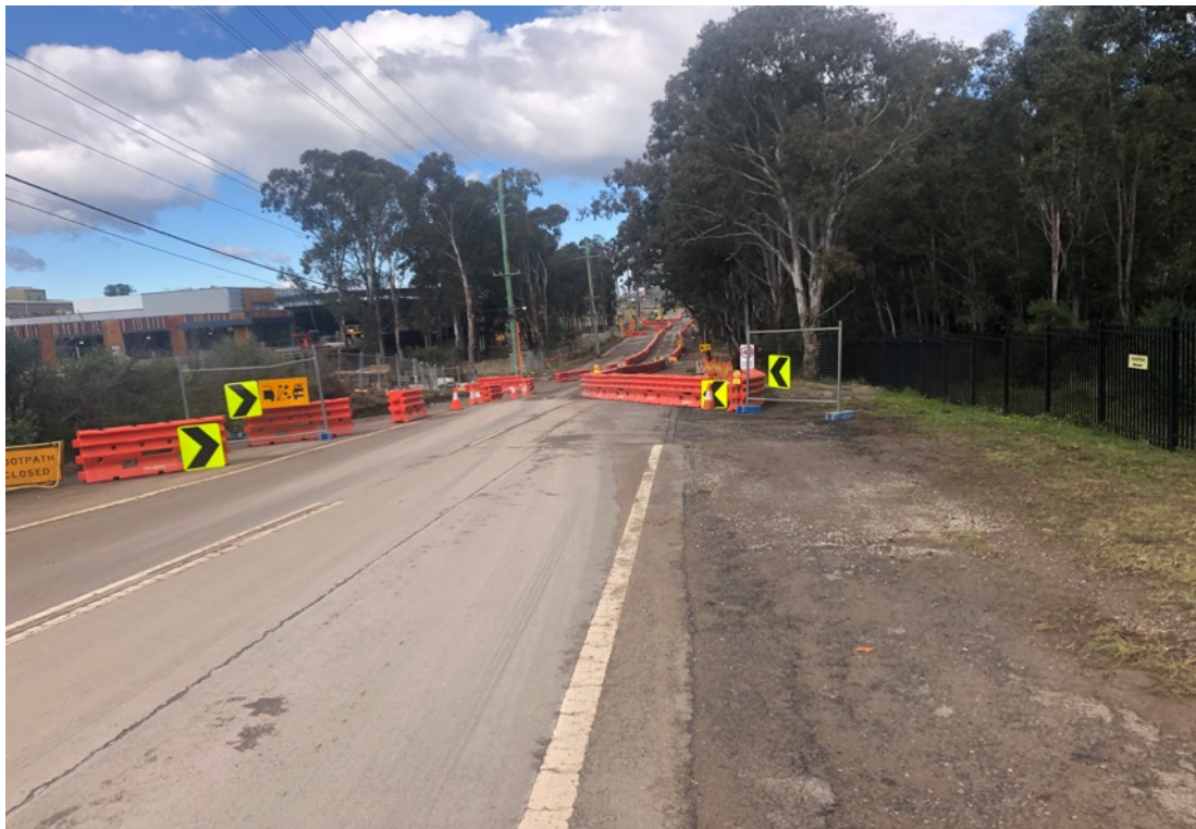
Photograph 3: Shows the existing streetscape along O'Connell St looking southwards
