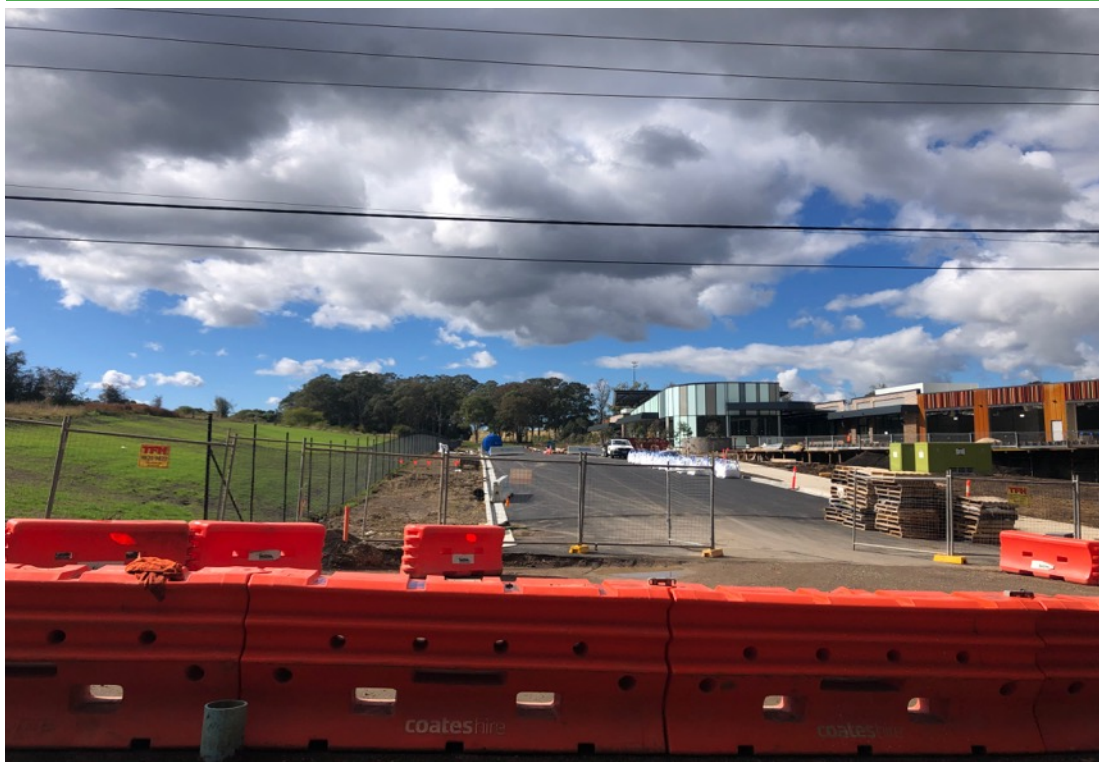
Photograph 4: Shows Caddens Corner, currently under construction which bounds the site's immediate southern boundary
