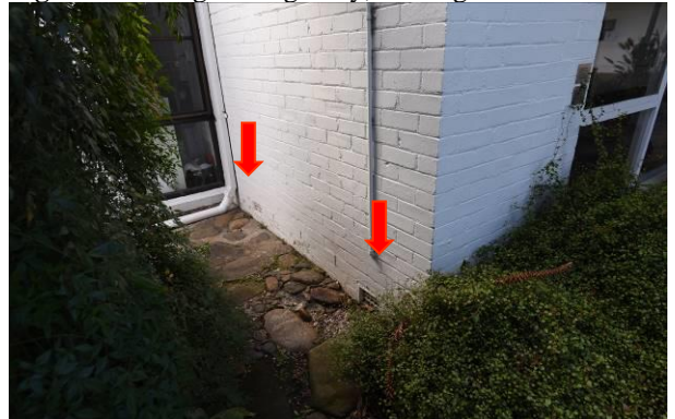
Figure 6: Existing ventilation grilles to northern wall of gallery.
