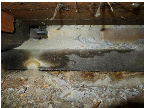
Figure 9: Evidence of fungal growth to bearers of Living Room Gallery subfloor.
