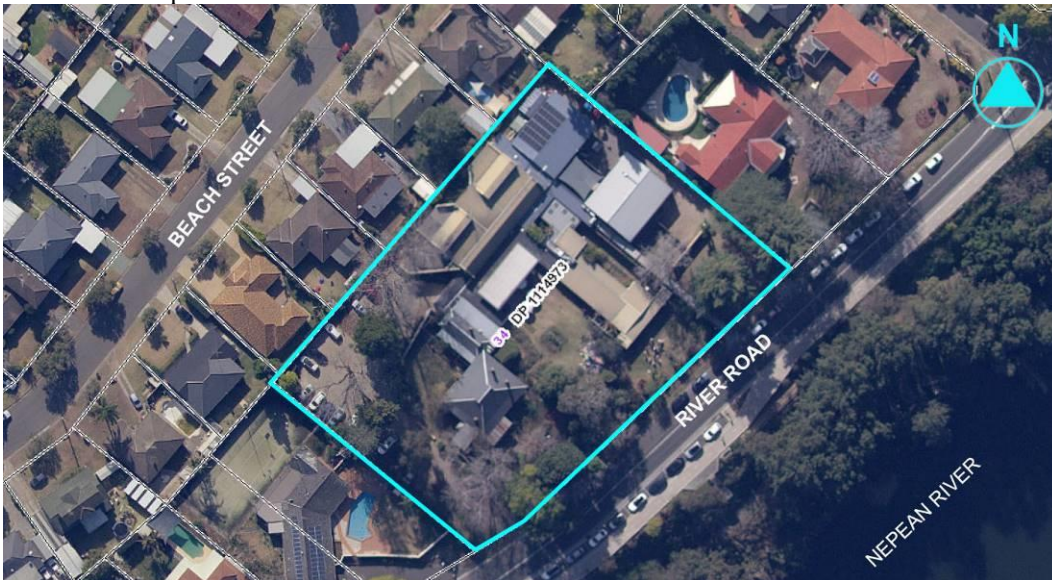
Figure 2: Aerial view of the subject property showing the legal allotment boundaries (outlined in blue). The real property definition is Lot 34, DP 1114973.
