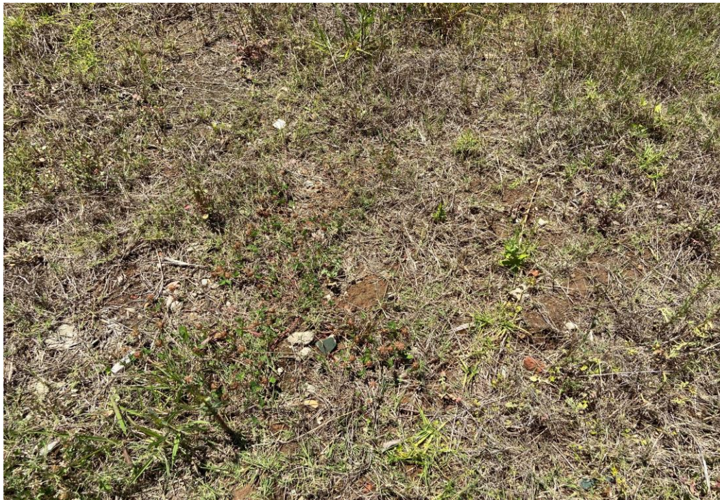
Photo 14 - Building/Demolition Waste (concrete) in the Grass on Number 30 (DP 2020)
