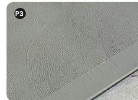
Plain grey broom finish concrete pavement for residential streetscape.
