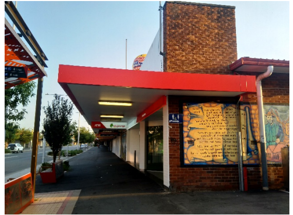
Figure 2 View looking north on Queen Street
