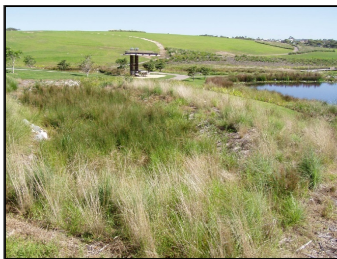
Plate 7-2 – Typical bio-retention system after plant establishment
