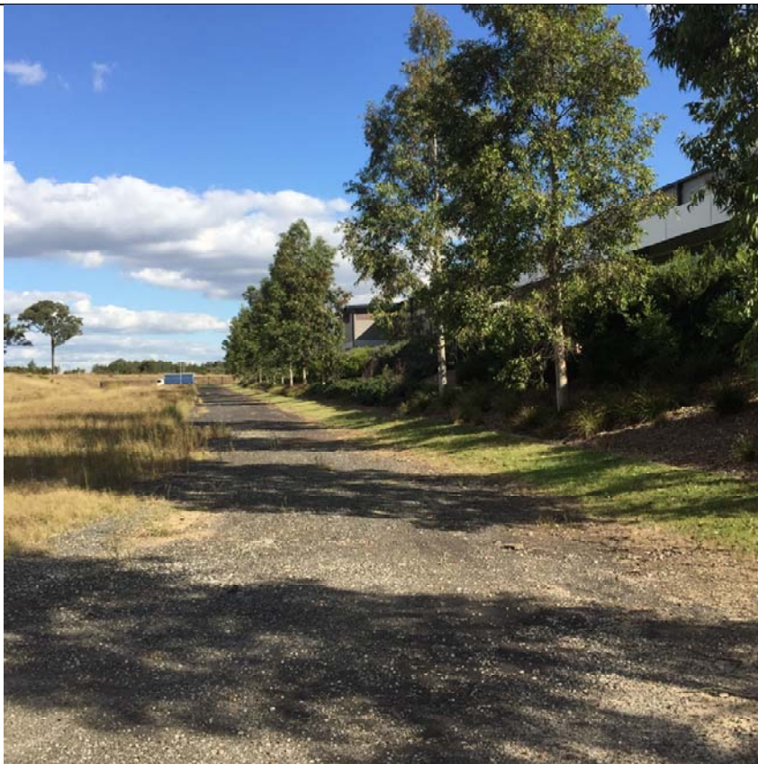
Site photo of proposed North-South Link Road location at approx. CH60 looking south.
