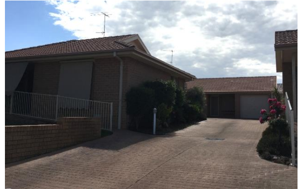
Figure 11 No. 68 Doonmore Street
