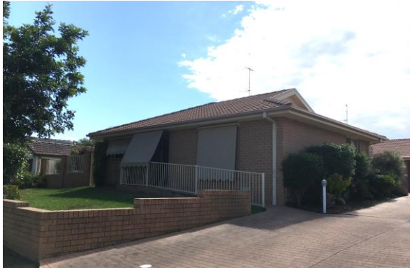
Figure 10 No. 68 Doonmore Street
