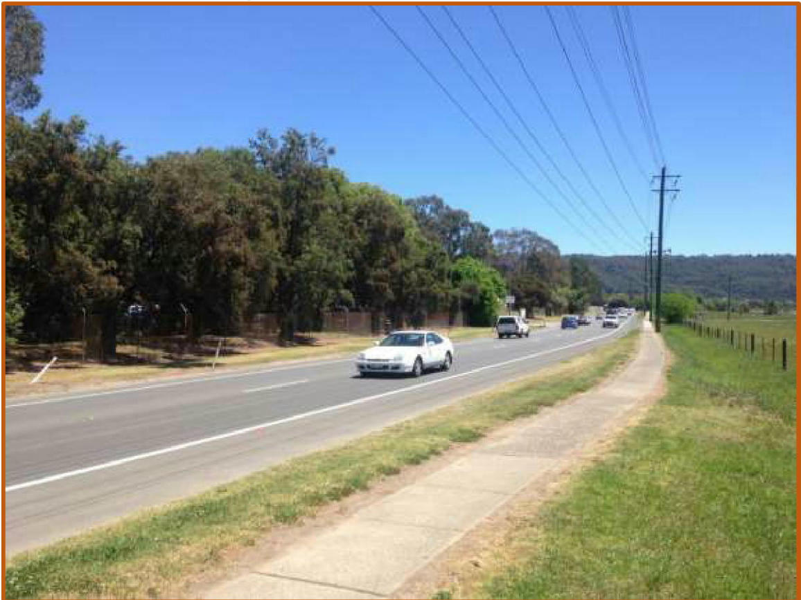
Photo 3: Looking west from ground level – adjacent to correctional centre entrance
