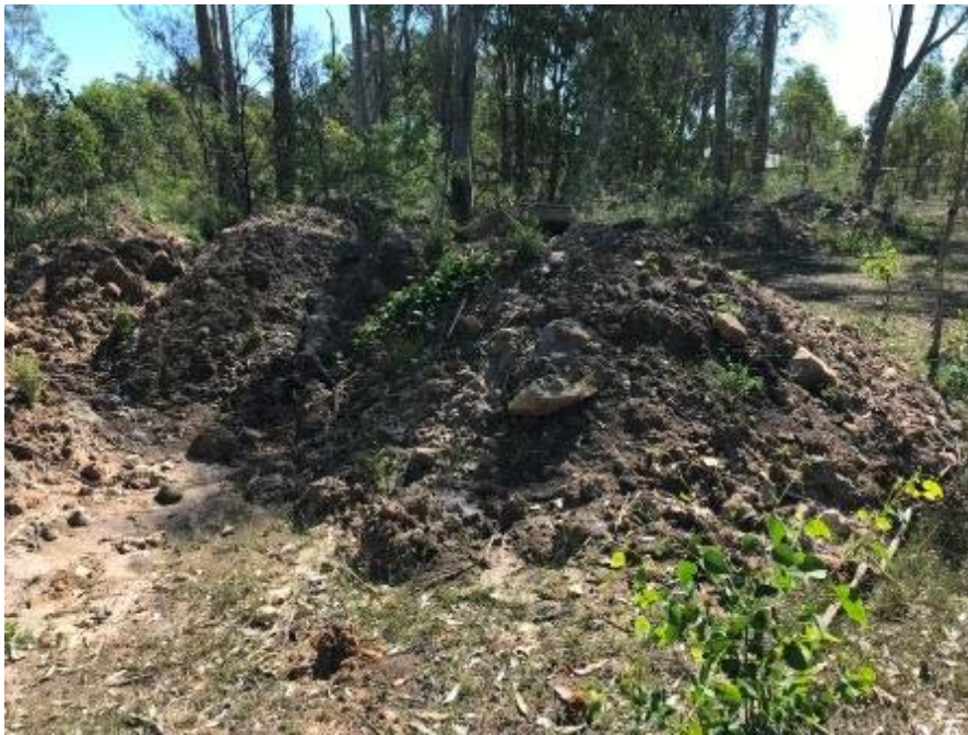
Image 6.8.5 View of stockpile SP05 adjacent to western boundary of the site
