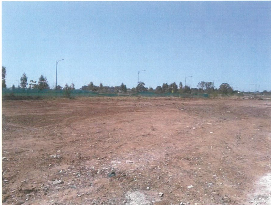
Photograph 7 - Filling in eastern portion of site
