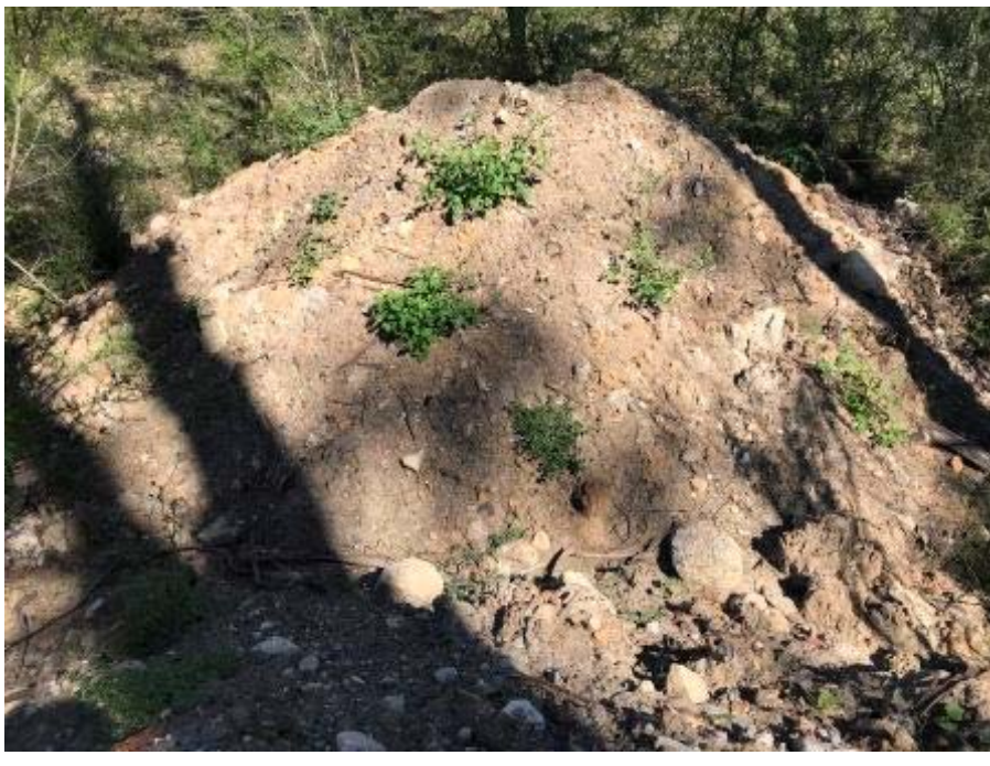
Image 6.8.8 View of stockpile SP08 adjacent to western boundary of the site
