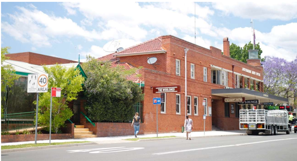
Figure 2: View of existing Beer Garden structure adjoining Hotel. Existing ramp, balustrade and steps to Beer Garden remain. No change proposed other than to planting.
