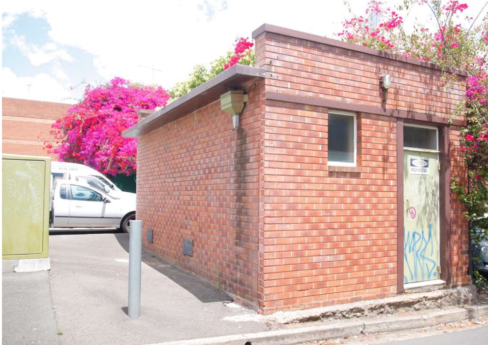
Figure 3: View of substation outbuilding on Lawson Lane. Parapet height proposed to be raised and new roof and improved roof drainage provided.
