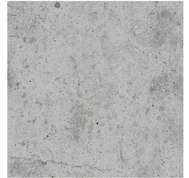
INSITU CONCRETE: Use: Custom Bench Seat Finish: Class Two
