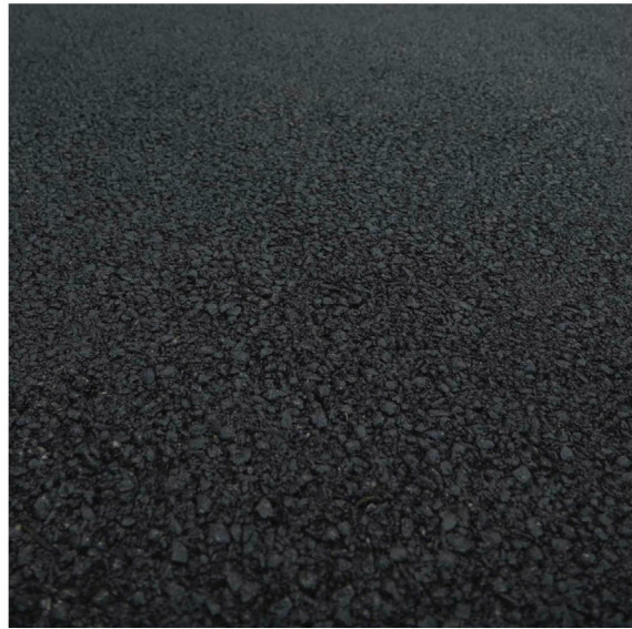
ASPHALT PAVING: Specification: 15mm AC5, Densely Graded on 35mm AC10 DGB20 Compacted sub-base to CBR4 - to match streetscape works
