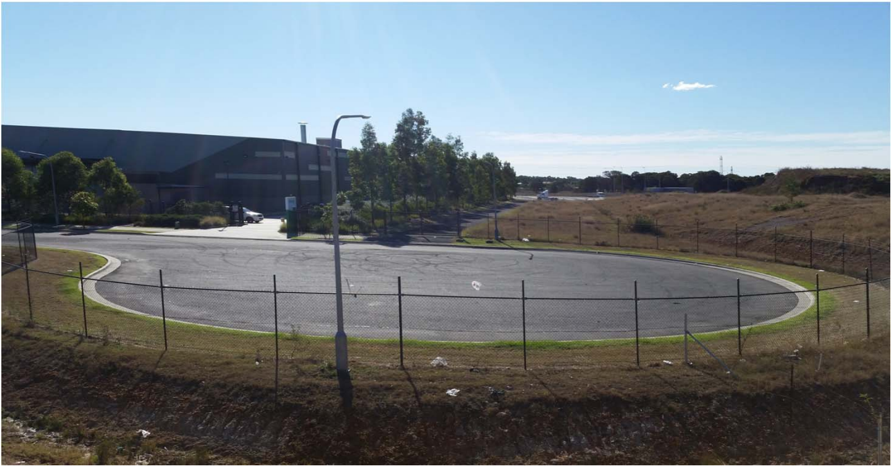
Photo 2- BH03 Looking South
