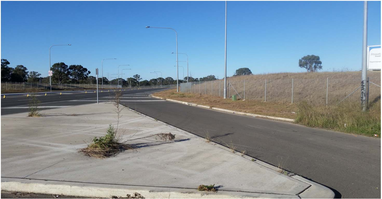
Photo 1- BH01 Looking East
