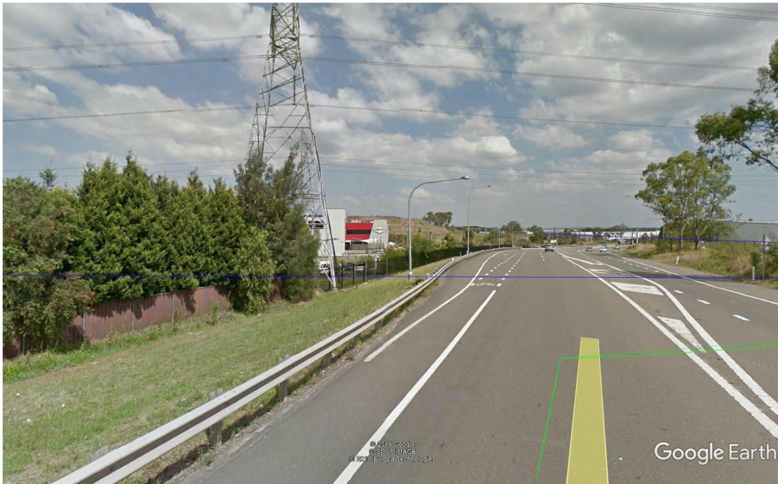
View of the site from the closest residential property to the north
