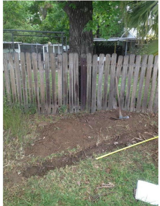
Figure 2: Part of the trench near T10.
