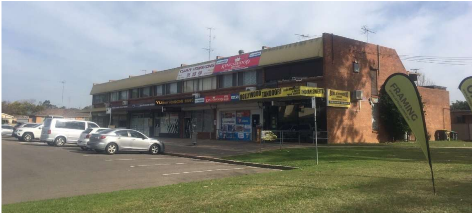
Figure 1.8: Neighbourhood shops, corner Manning Street and Second Avenue.
