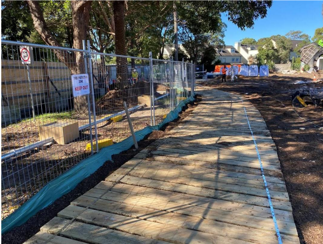
Figure 5. Example of tree protection fencing and ground protection.
