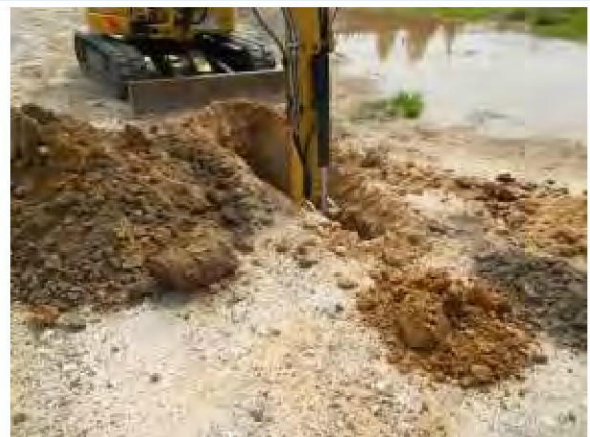
Photo 6. Fill and natural soils stockpiled adjacent test pit.
