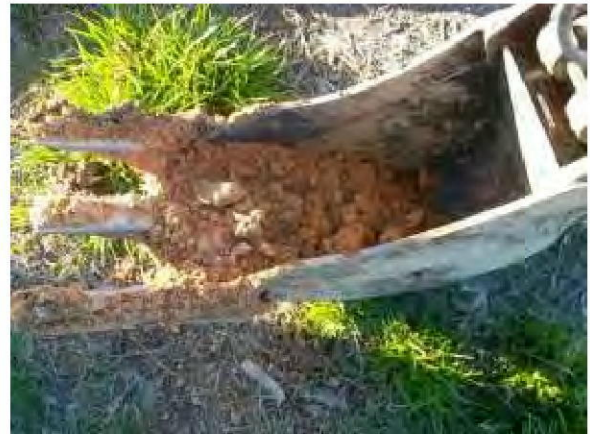
Photo 4. Natural soil within the bucket of the excavator.
