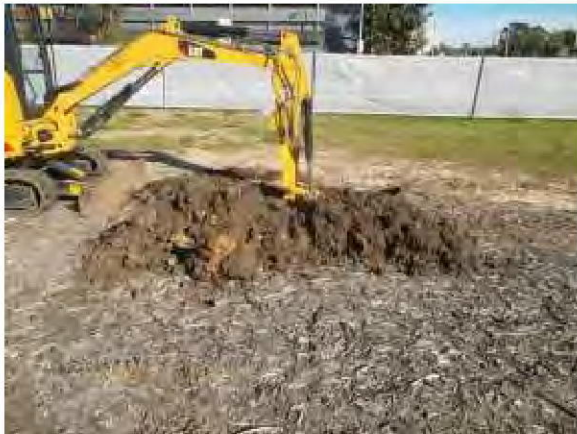
Photo 3. Fill stockpiled adjacent test pit..
