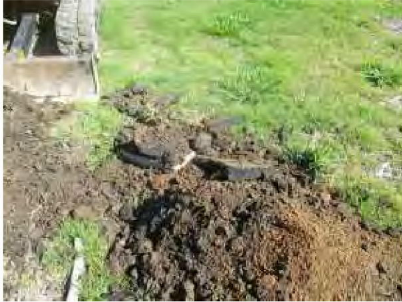
Photo 7. Bitumen excavated at approximately 0.3 m BGL at TP17, TP 18 and TP19.
