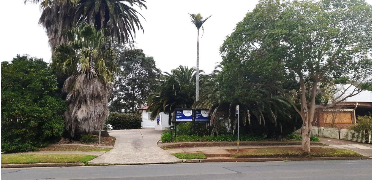
Figure 2 Site frontage viewed from Derby Street
