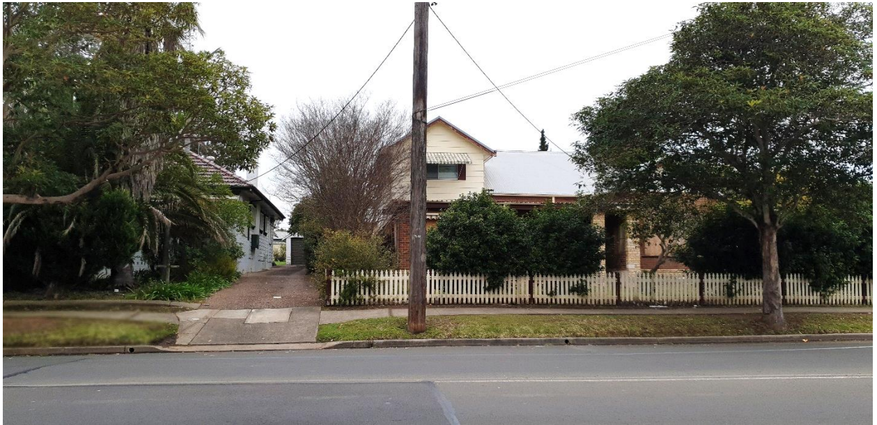
Figure 8 No. 172 Derby Street (adjoining site to the west)
