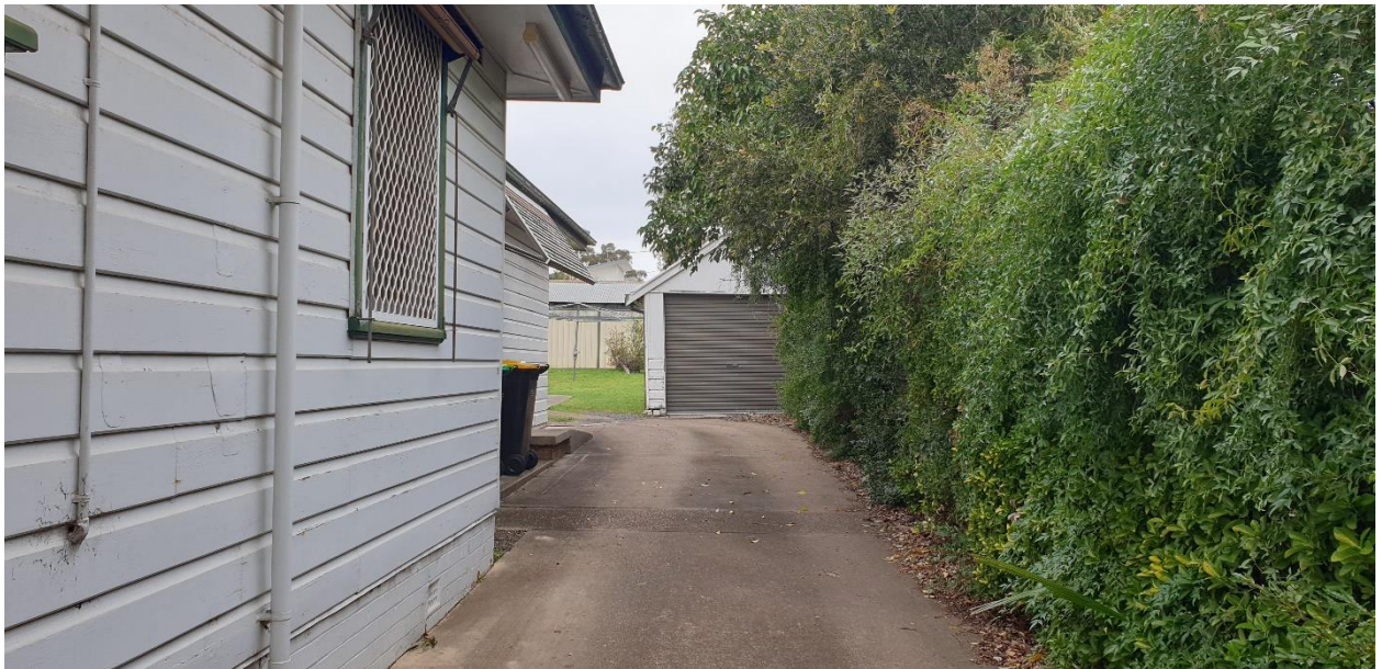
Figure 5 Garage located to the rear of site south of existing single storey building
