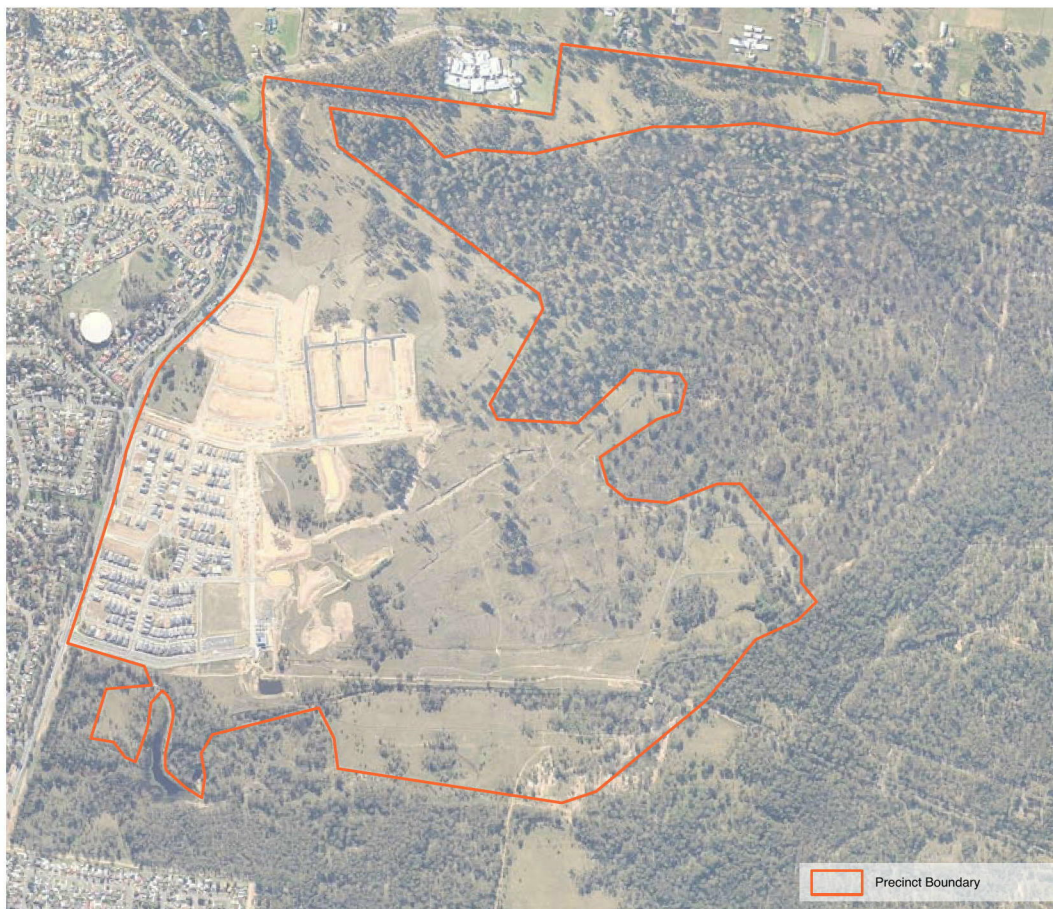
Figure 1.3 Aerial View: Western Precinct Works Area
