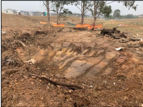
Photo 1: 08 January 2020: Commencement of excavation in remediation zone.
