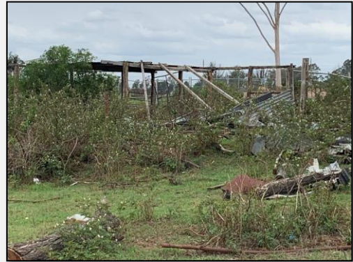
Photo 10: 05 February 2020: Inspection of secondary remediation area prior to remediation works.
