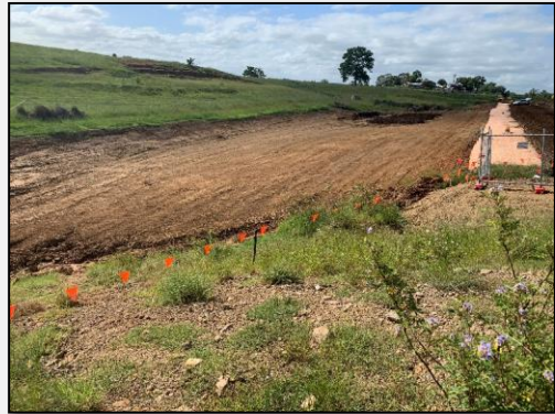
Photo 22: 23 March 2020: Remediation area has been graded to control surface water flows.
