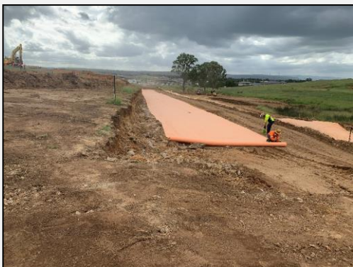
Photo 23: 23 March 2020: Geofabric being placed over cell.
