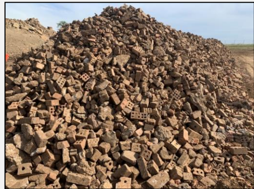
Photo 14: 28 February 2020: Stockpiled screened oversize segregated in preparation for pulverising.
