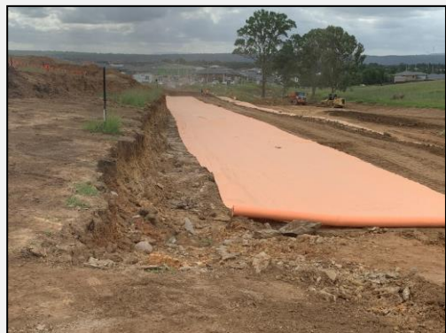
Photo 24: 23 March 2020: Geofabric being placed over cell.
