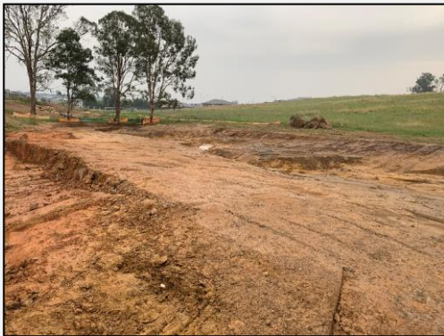
Photo 3: 24 January 2020: Completion of excavation in remediation zone.
