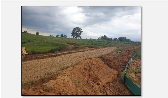
Photo 26: 25 March 2020: Capping completed over cell.
