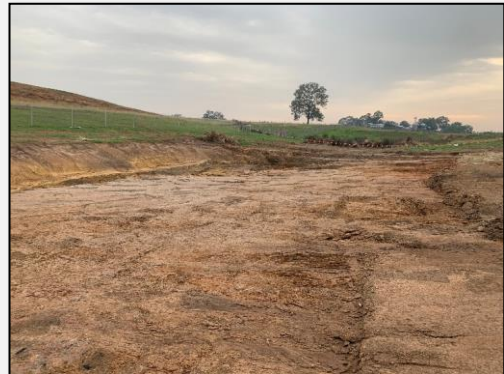
Photo 4: 24 January 2020: Completion of excavation in remediation zone.
