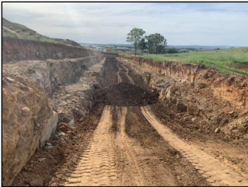
Photo 15: 28 February 2020: Containment cell. Stockpile of waste awaiting spreading and compaction.
