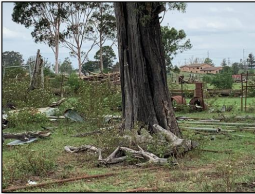
Photo 9: 05 February 2020: Inspection of secondary remediation area prior to remediation works.
