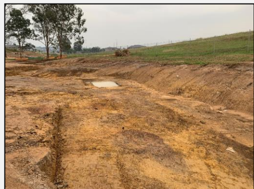
Photo 6: 24 January 2020: Completion of excavation in remediation zone.
