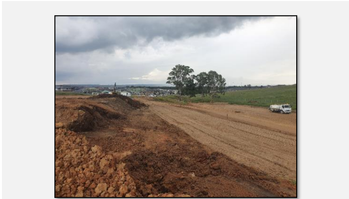
Photo 25: 25 March 2020: Capping completed over cell.
