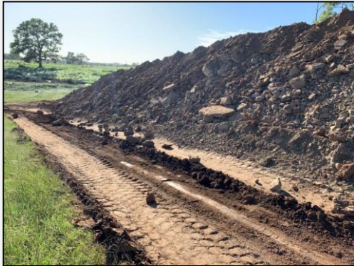
Photo 13: 28 February 2020: Stockpiled VENM adjacent to treatment area.
