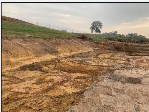
Photo 5: 24 January 2020: Completion of excavation in remediation zone.
