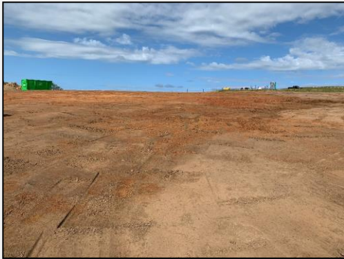
Photo 19: 23 March 2020: Treatment/stockpiling area post completion of cell.
