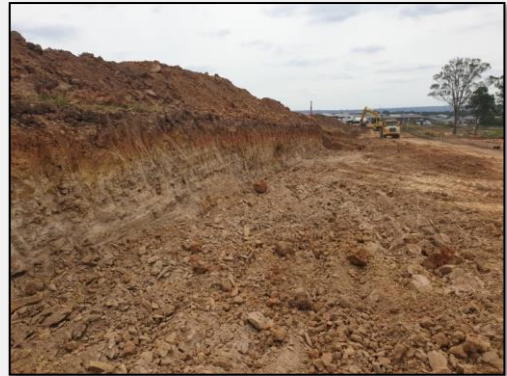
Photo 8: 05 February 2020: Commencement of containment cell construction.
