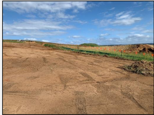
Photo 20: 23 March 2020: Treatment/stockpiling area post completion of cell.
