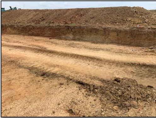
Photo 7: 05 February 2020: Commencement of containment cell construction.
