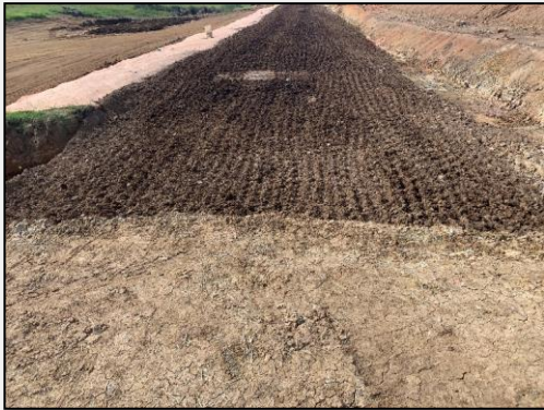
Photo 21: 23 March 2020: Completion of cell, geofabric placed on lower edge.
