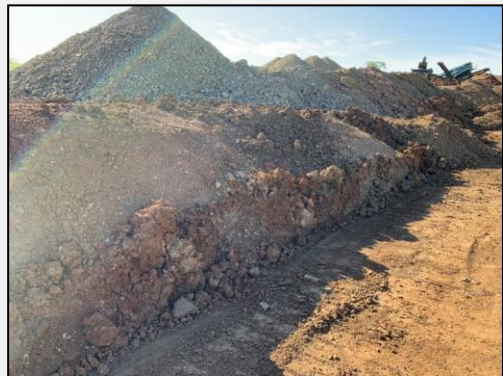
Photo 16: 28 February 2020: Stockpiled VENM adjacent to treatment area.
