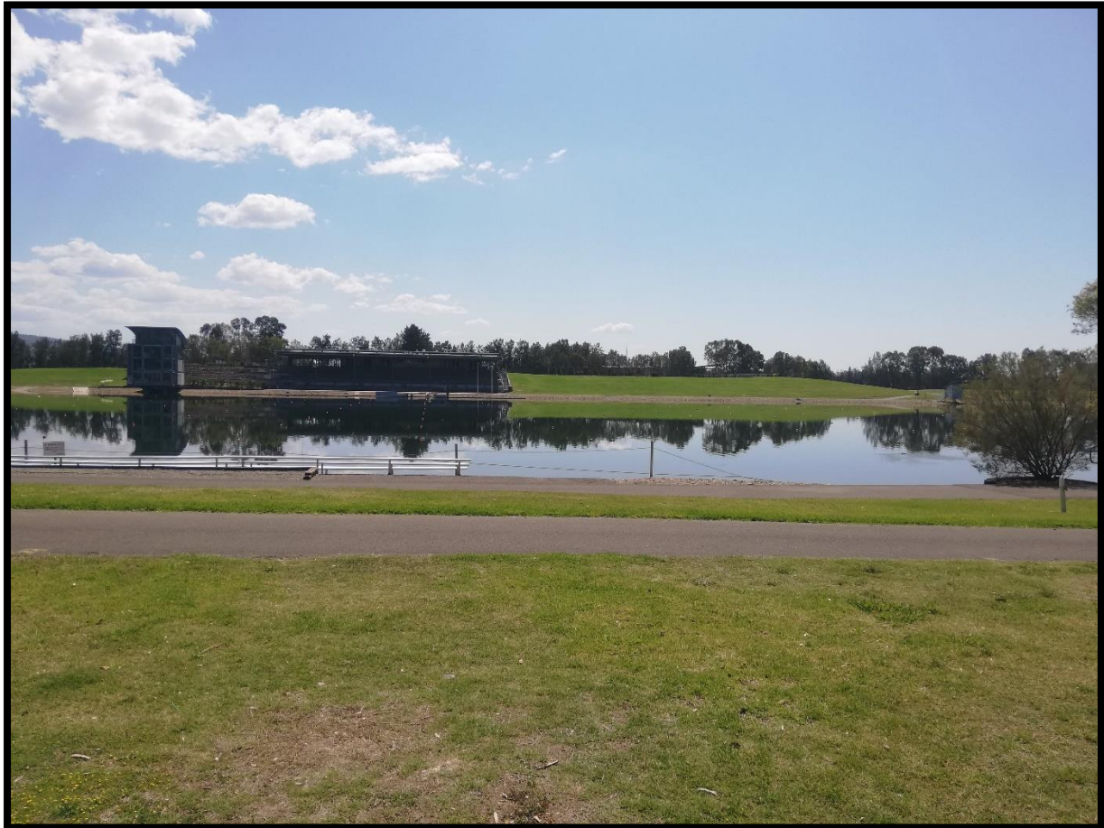
Figure 15: Pole Smart Pole SC2Location – Looking North
