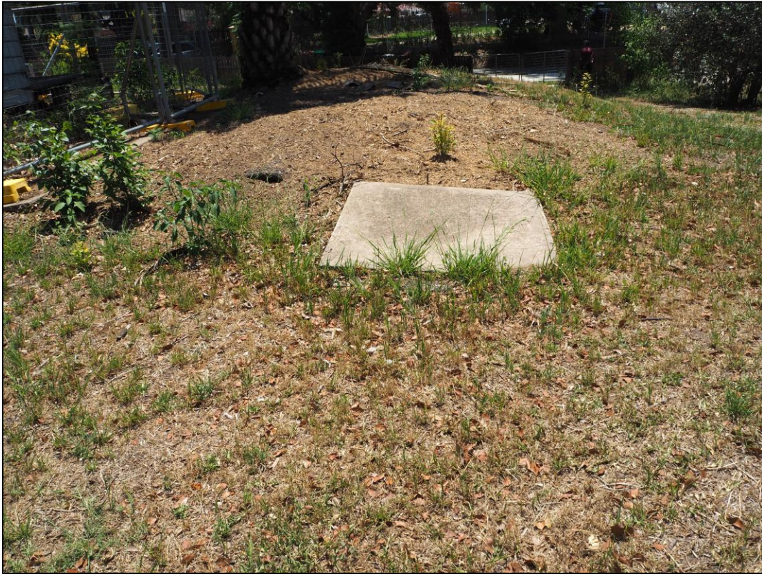
Photograph 5: Showing a small extant concrete slab at the rear of the study area.
