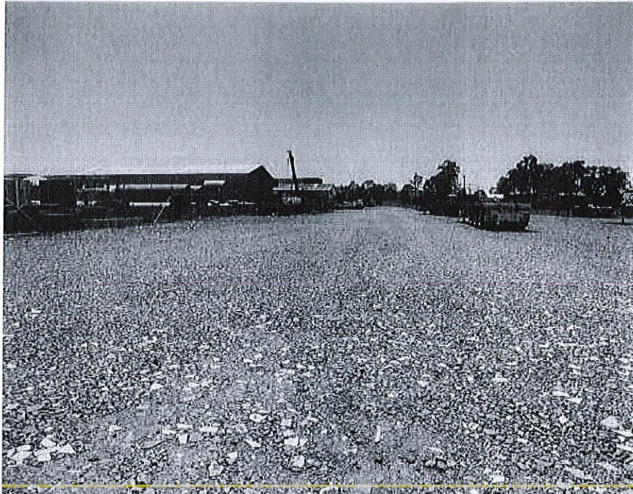
A: Site Condition – taken within south western portion of the site, looking east
