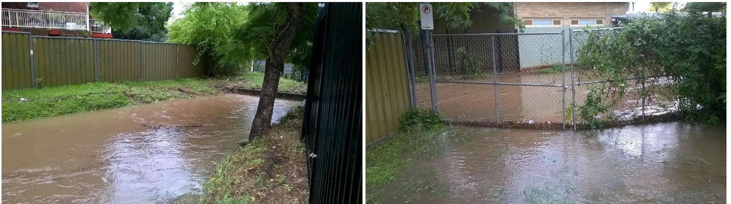
Figure 3-4 Flow within the adjacent channel (Left) Upstream of the channel with flow entering from a culvert under Station St (Right) Flow from the channel into Station Lane
