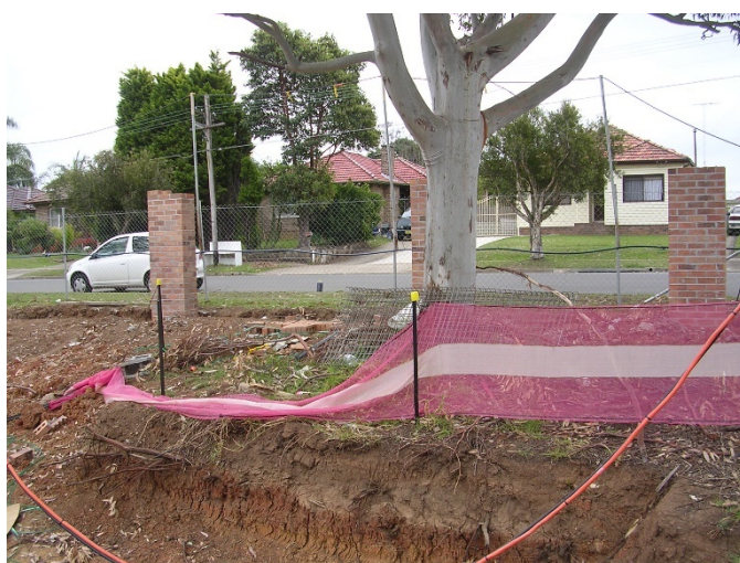
Photo 6: Woven fences seldom work particularly when space is limited.
