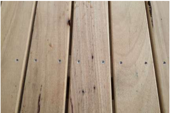
Blackbutt or similar / 75mm x 18mm External Cladding & Garage Ground Floor
