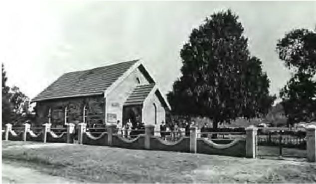
Figure 2.9 Northern elevation of Emu Plains former Methodist Church, c1930s
