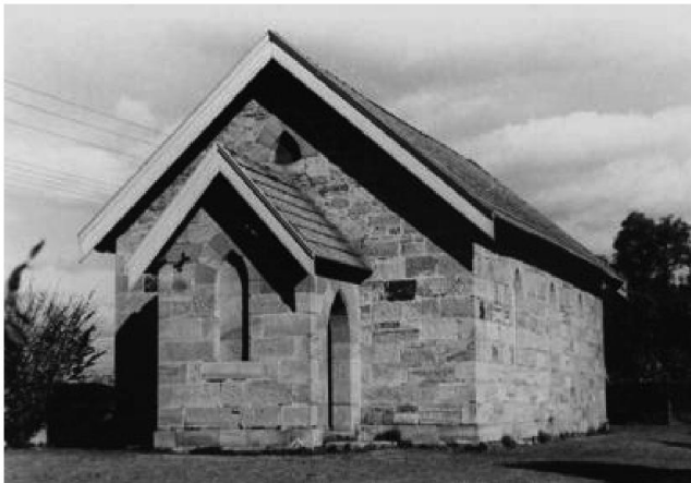
Figure 2.10 Northern elevation of Emu Plains former Methodist Church, date unknown. This elevation shows the small porch with two entrances and a blind arch. This arrangement has not changed
