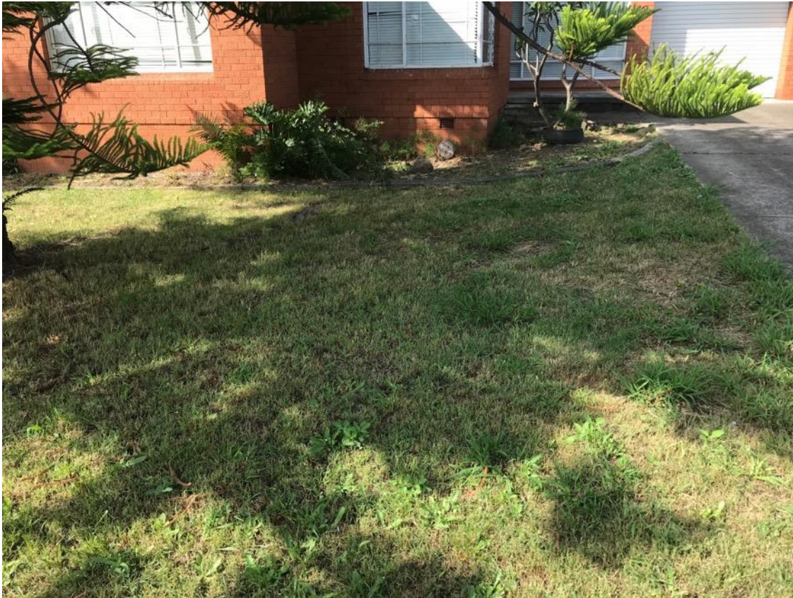
Figure 8. South facing view of 76 Hobart Street, St Marys, including healthy grass coverage, small and medium plants, partial view of the concrete driveway and single storey brick residential building.
