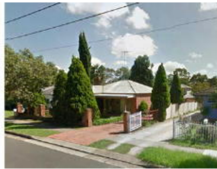
Derby Street dual occupancy development to the east
