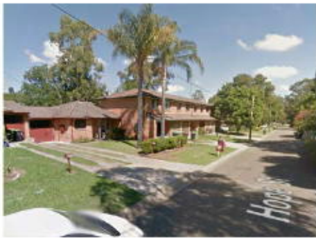
Department of Housing development to the north on Hope Street
