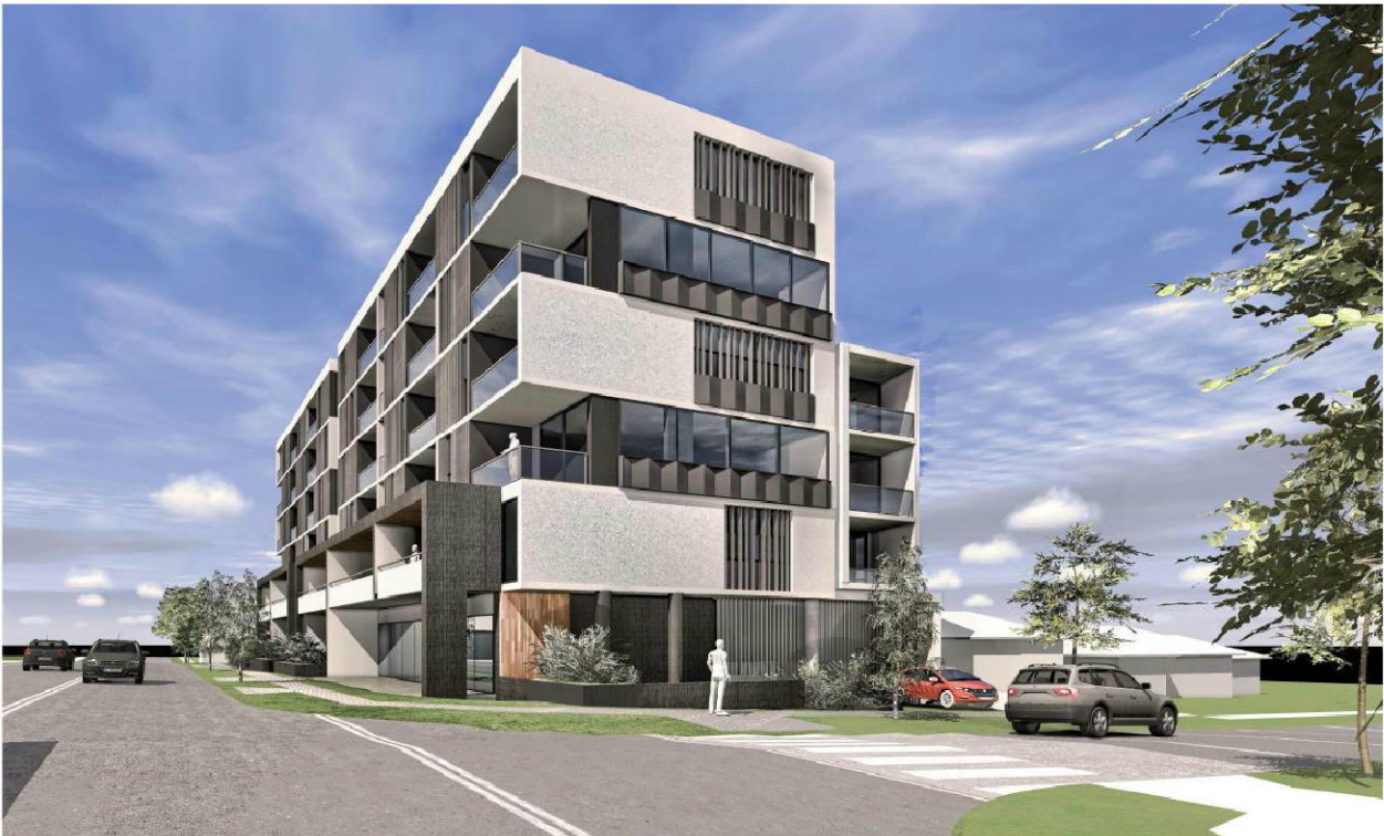
PICTURE 7 – LOOKING NORTH UP SOMERSET STREET
