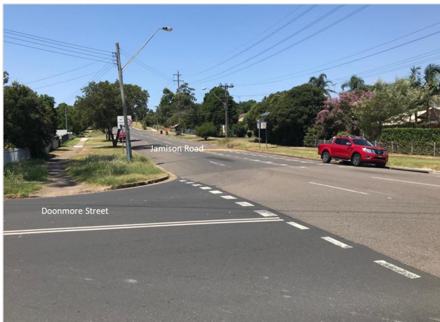
Figure 2-5: View looking east on Jamison Road and Doonmore Street intersection
