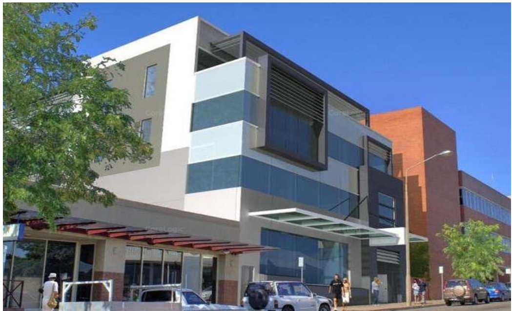
331 High Street view to the north-east of the High Street frontage.
