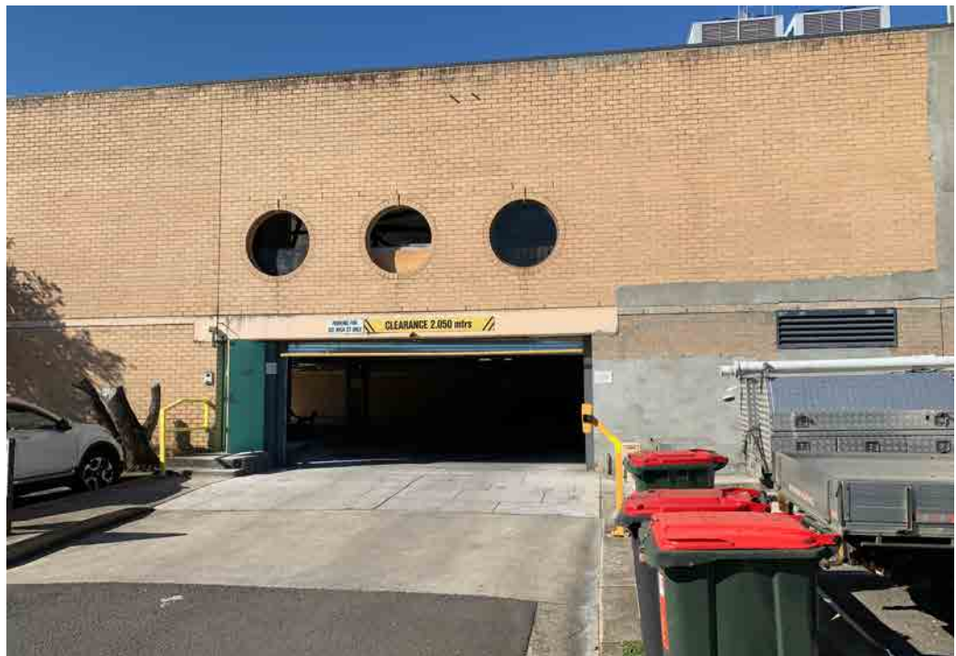
View west on Lawson Lane
