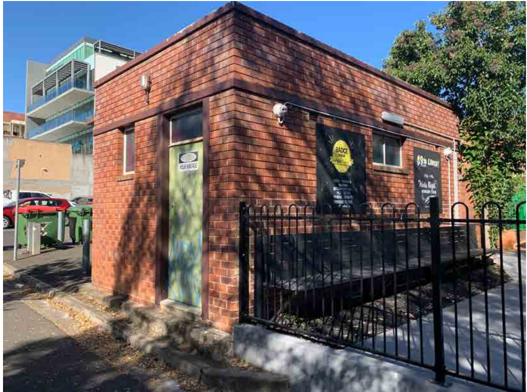
View of the substation from Lawson Lane
