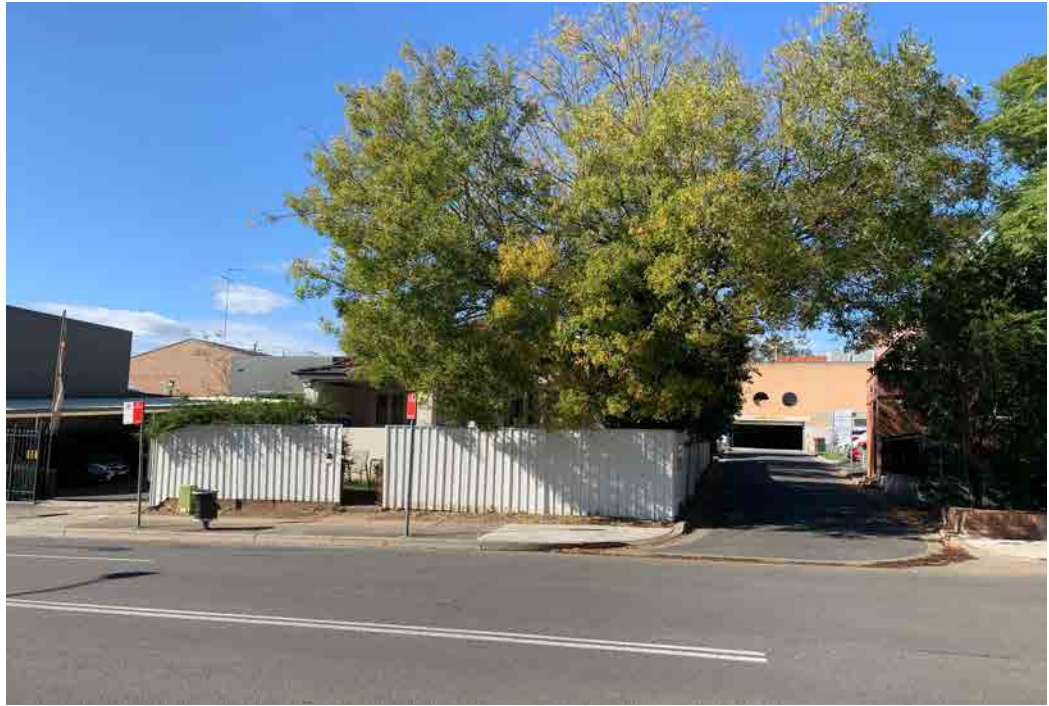
View east of the subject site 18 Lawson Street and Lawson Lane from Edwards Place
