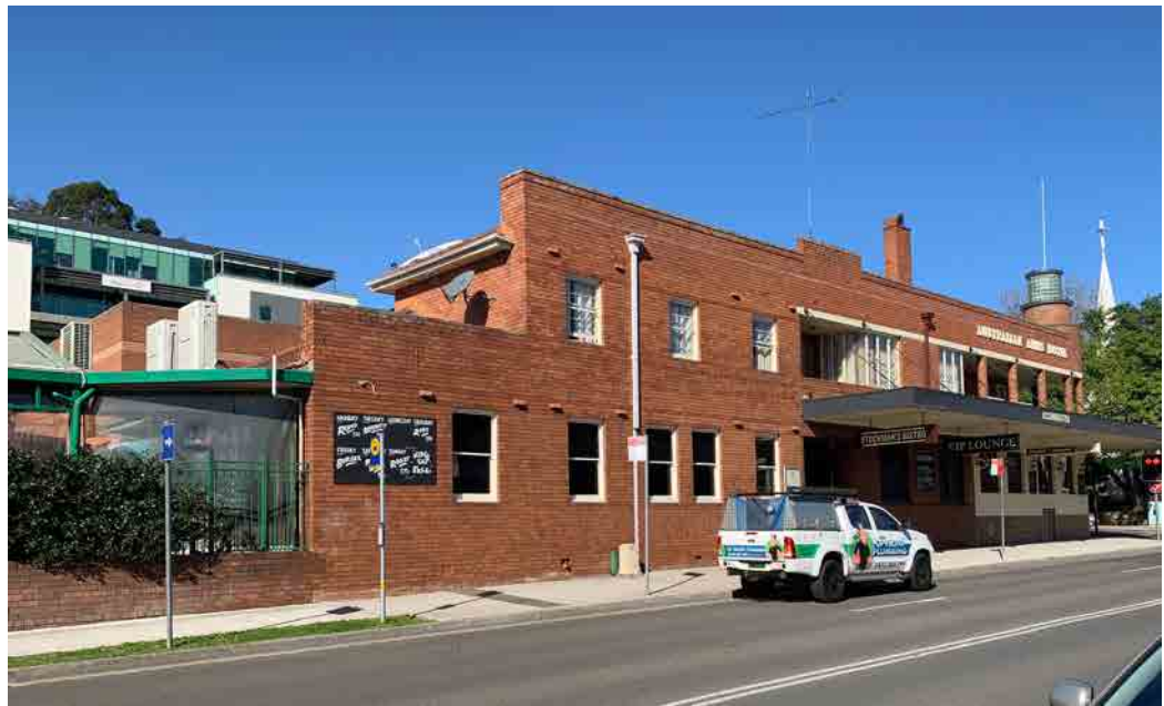
Covered beer garden on north-west of the site interface with Hotel
