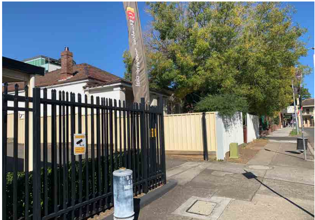
View south of the subject site 18 Lawson Street from Lawson Street
