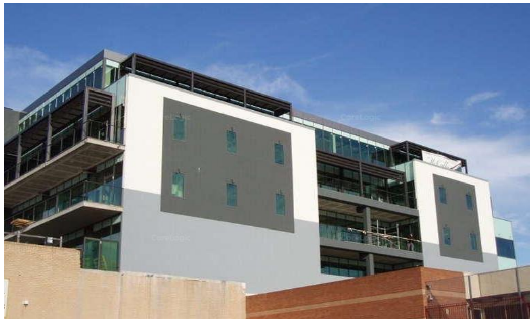
331 High Street view to the south-east adjoining the eastern boundary.
