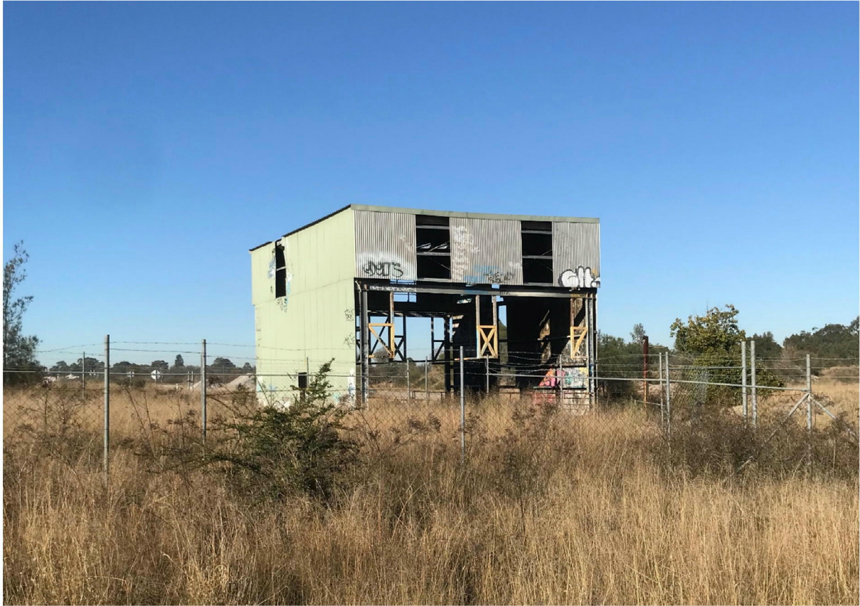
Figure 2 – Disused Dump Station Shed (Photo 1)
