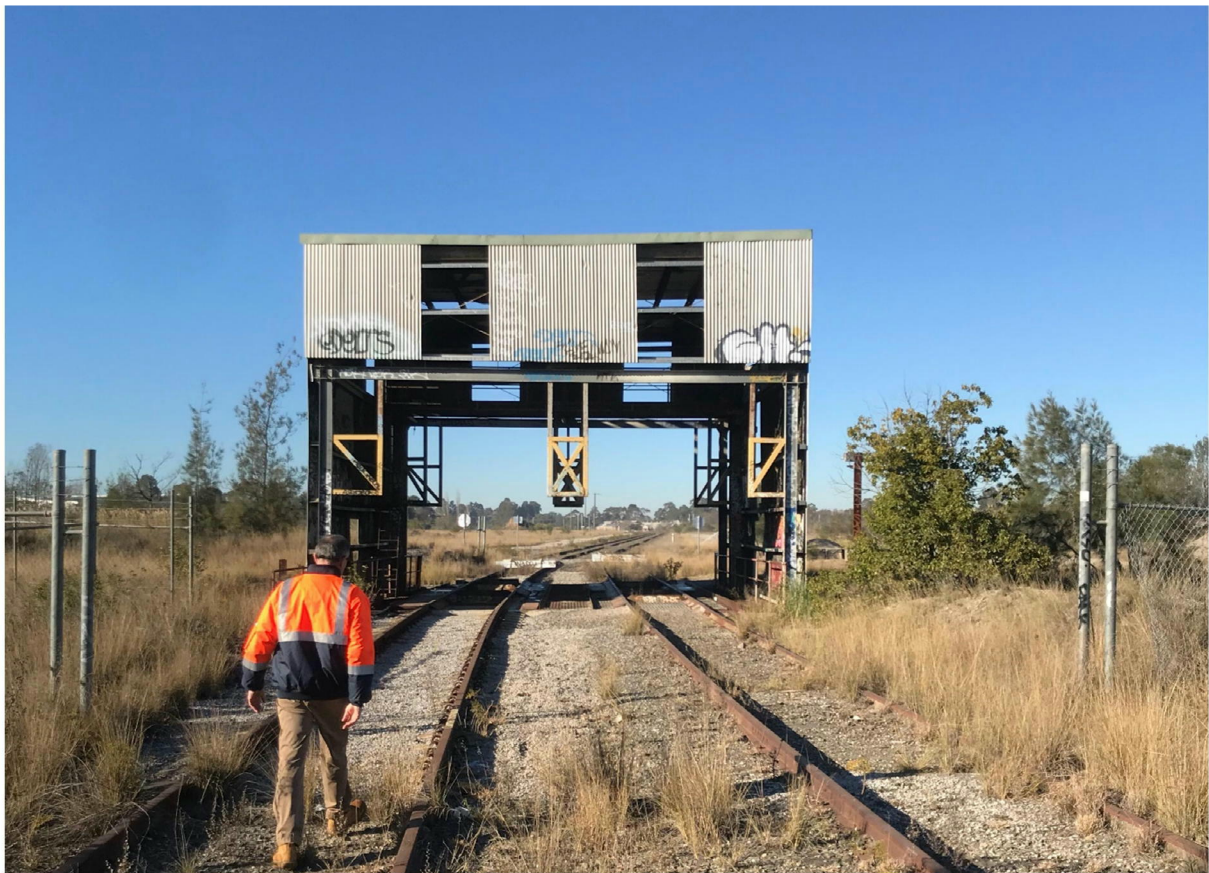
Figure 3 – Disused Dump Station Shed (Photo 2)
