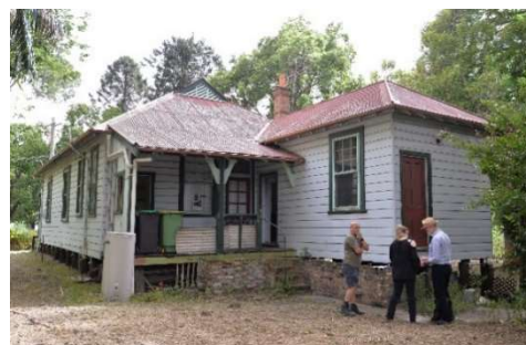
Figure 6: Southern (rear) elevation of former Police Station Building.
