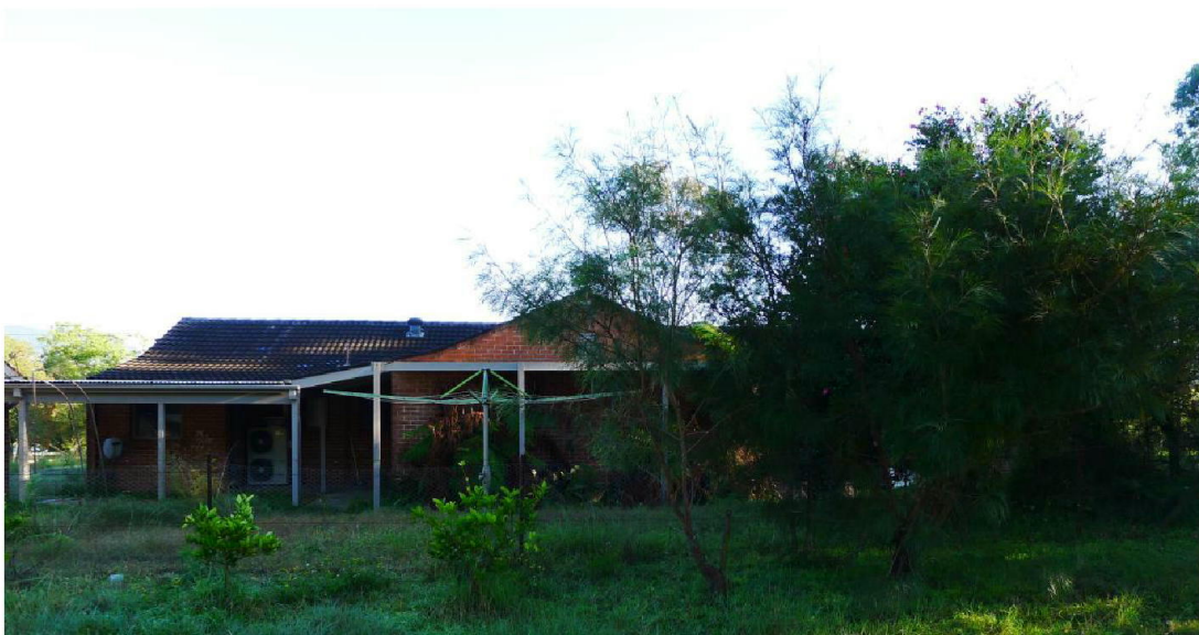
Photo 6 – The existing house
