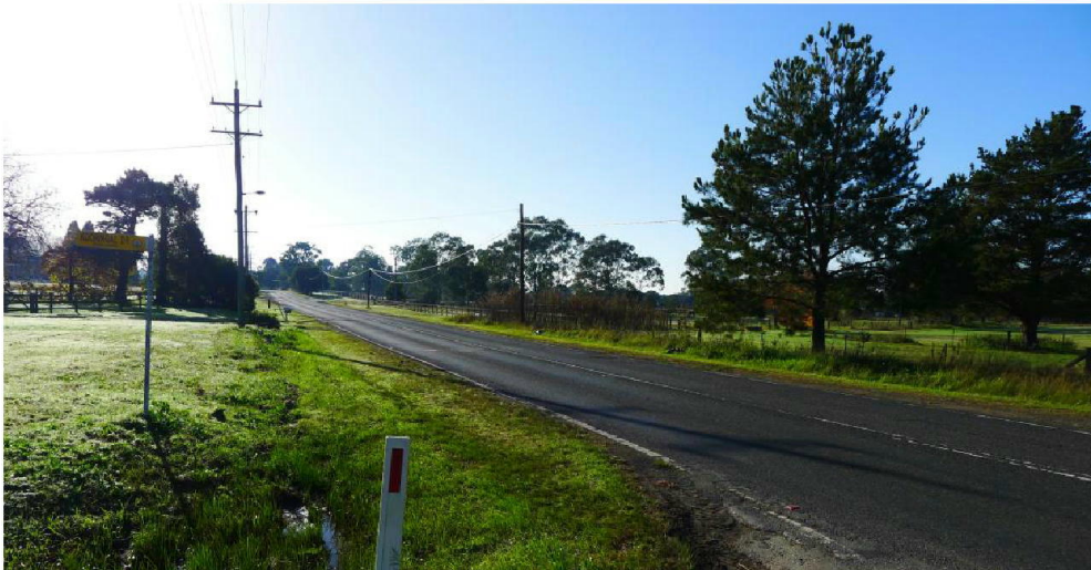
Photo 2 – Castlereagh Road looking northeast
