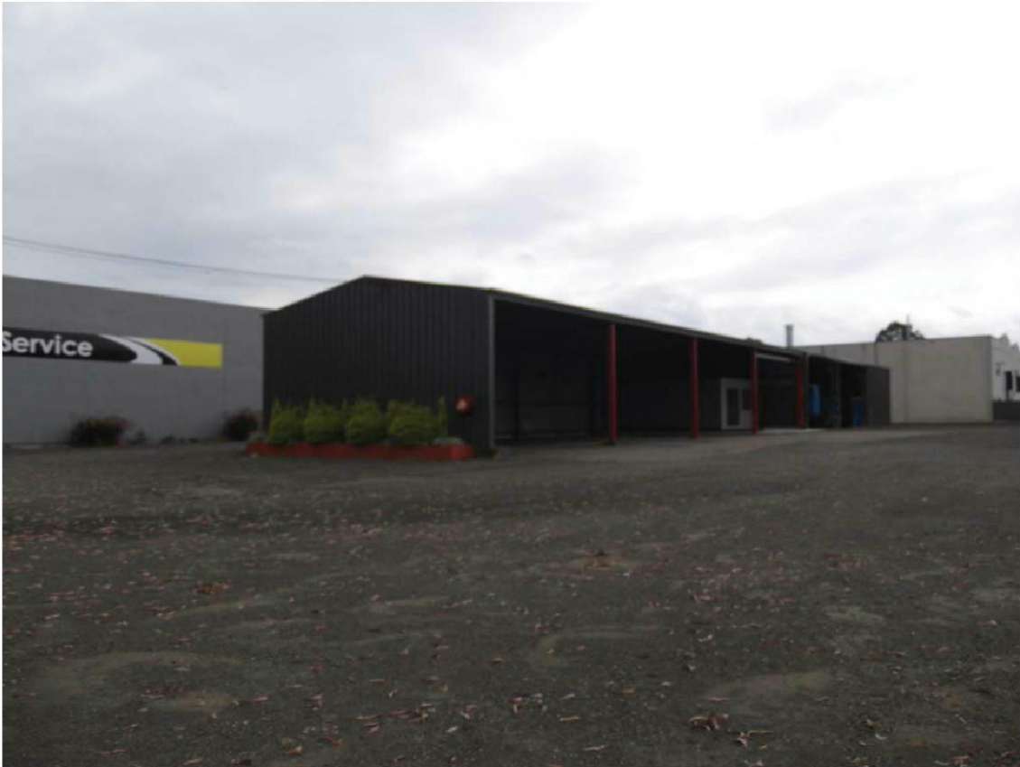
Photo 1: The front of the shed looking south west
