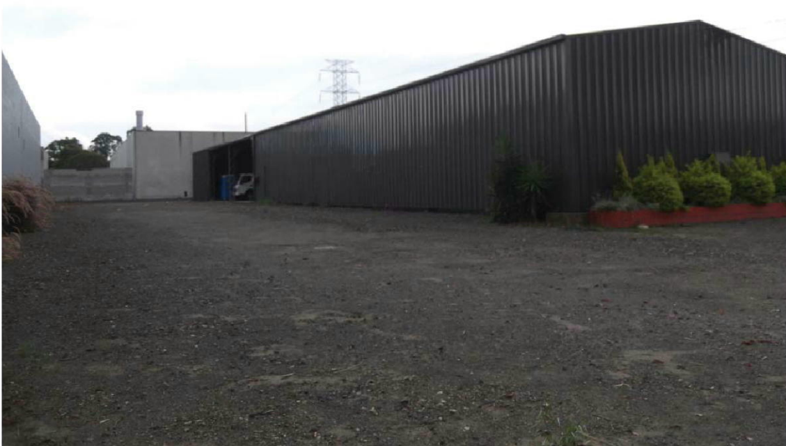
Photo 4: Rear of the shed looking north west
