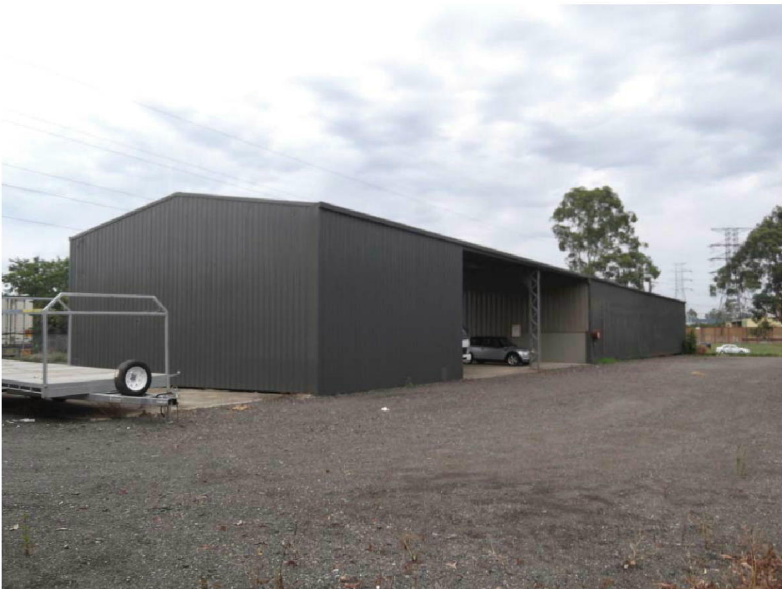
Photo 2: The rear of the shed looking north east
