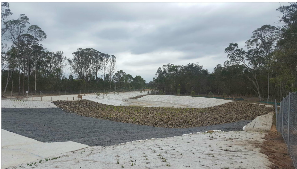
Photograph 3: Stormwater basin and perimeter maintenance road along southern interface
